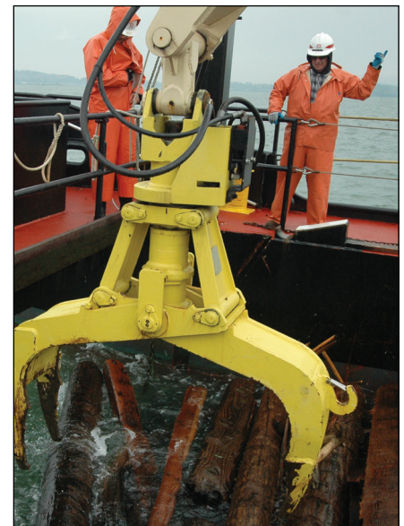
Raccoon crewmembers gather debris using the boat's powerful hydraulic crane.
